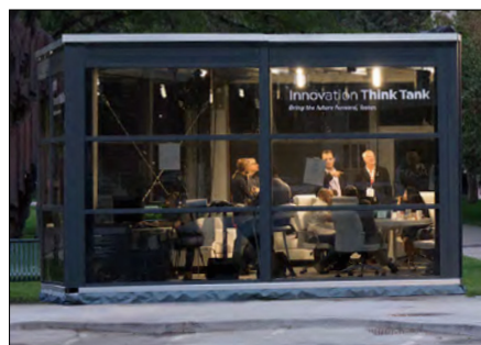
The glass Think Tank physically reinforced the client’s position as a forward-thinker, challenging the convention of brick-and-mortar with a transparent structure that made discussions visible and better integrated within the broader community.
